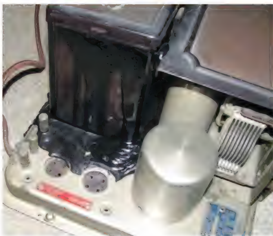
This radio had shorted filter capacitors in the power supply which caused overcurrent, overheating, and melting in the power transformer.
